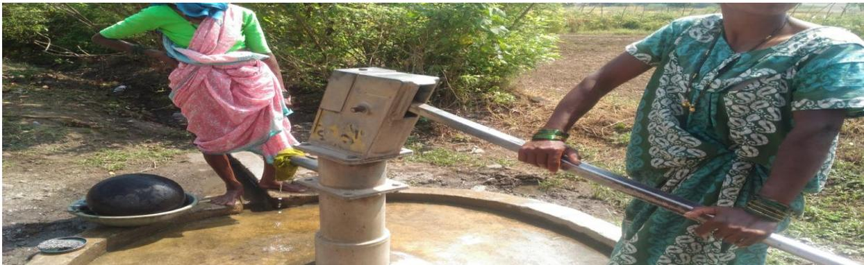
Figure 3 - Women taking water using hand pumps. The mouth of the pump is covered with cloth that to filter the water that comes out with red sediments
